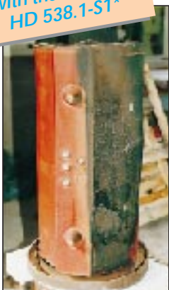
Trihal transformer coil after the test F1.
