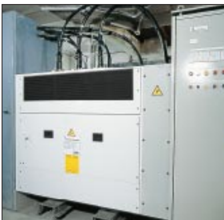
(1) by removing dismantled panels of the enclosure.
