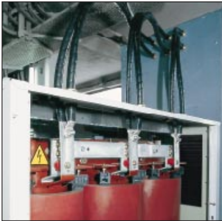
HV connections from above with plug-in connectors (1) (option).
