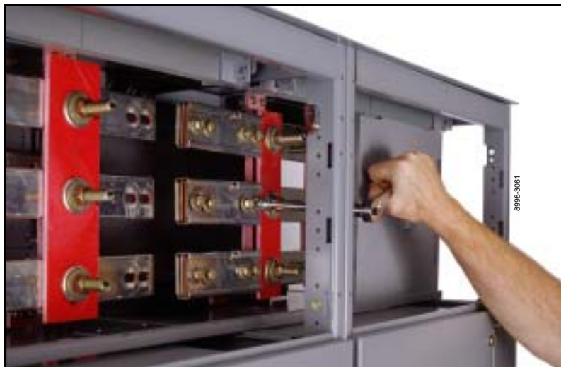
Figure 14: Removing the Bolts on the Splice Assembly
