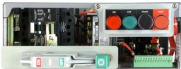
Figure 36: Operator Handle in the OFF Position
