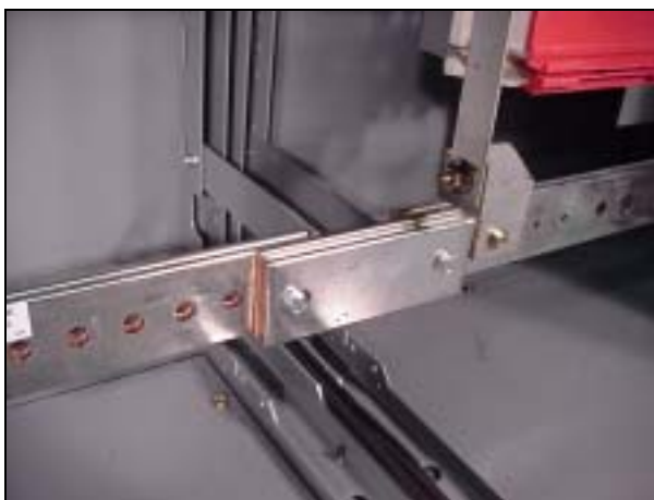
Figure 19: Ground Bar Bolts Replaced
