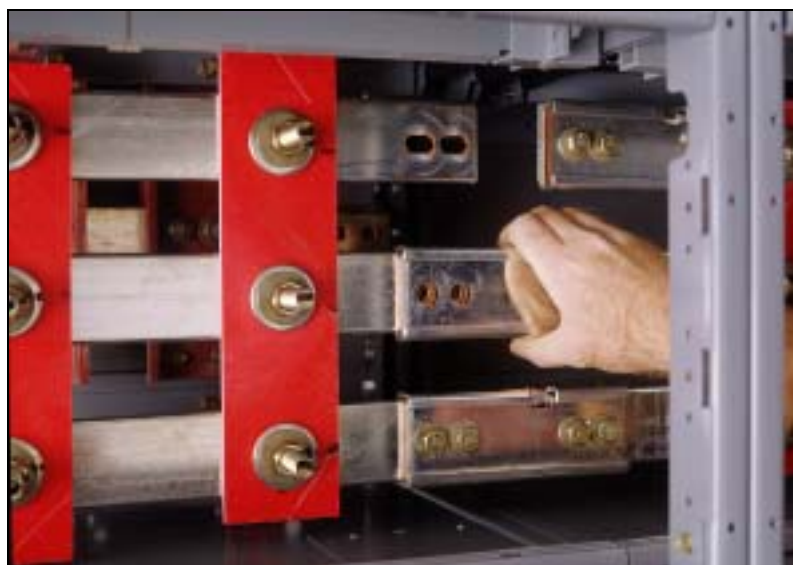
Figure 15: Aligning the Splice and Bus Holes
