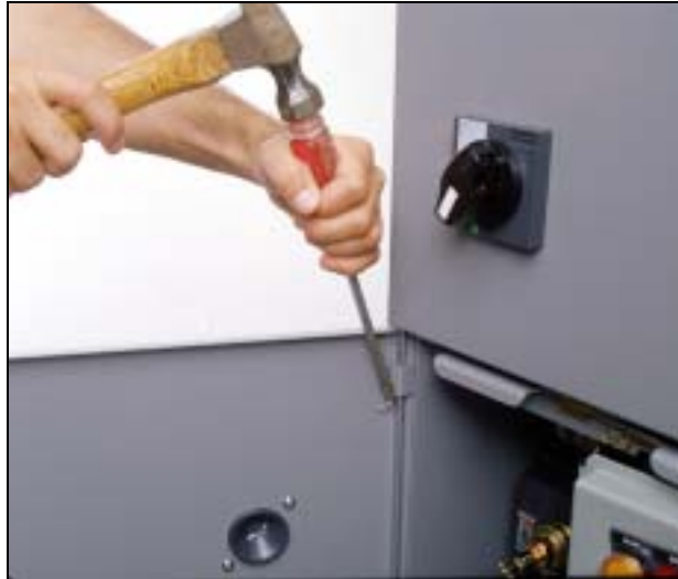
Figure 35: Driving Out the Hinge Pin
