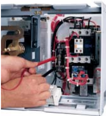
Figure 41: Inspecting Fuses
