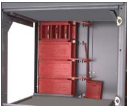
Figura 44: Persiana del bus vertical manual
