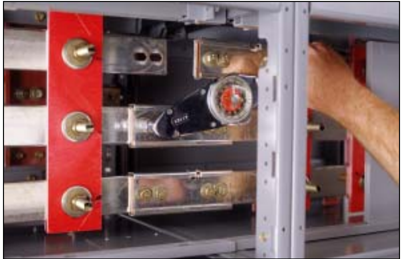
Figure 17: Torquing the Bolts
