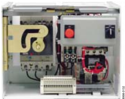
Figure 49: Handles Flush with the Front of the MCC
